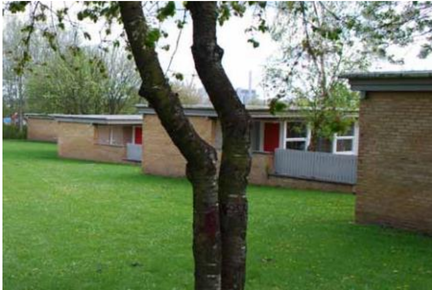
Figure 14. Photo of the single-family houses with flat roofs, poor thermal insulation in façades and gables, as well as many thermal bridges in the building envelope. Photo: Ole Balslev-Olesen.
